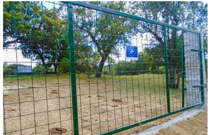
Fig. 6 Fencing to protect sheep and cattle from wolves, constructed from iron mesh welded panels, cement and granite poles and a concrete plinth under the gates to prevent digging.
